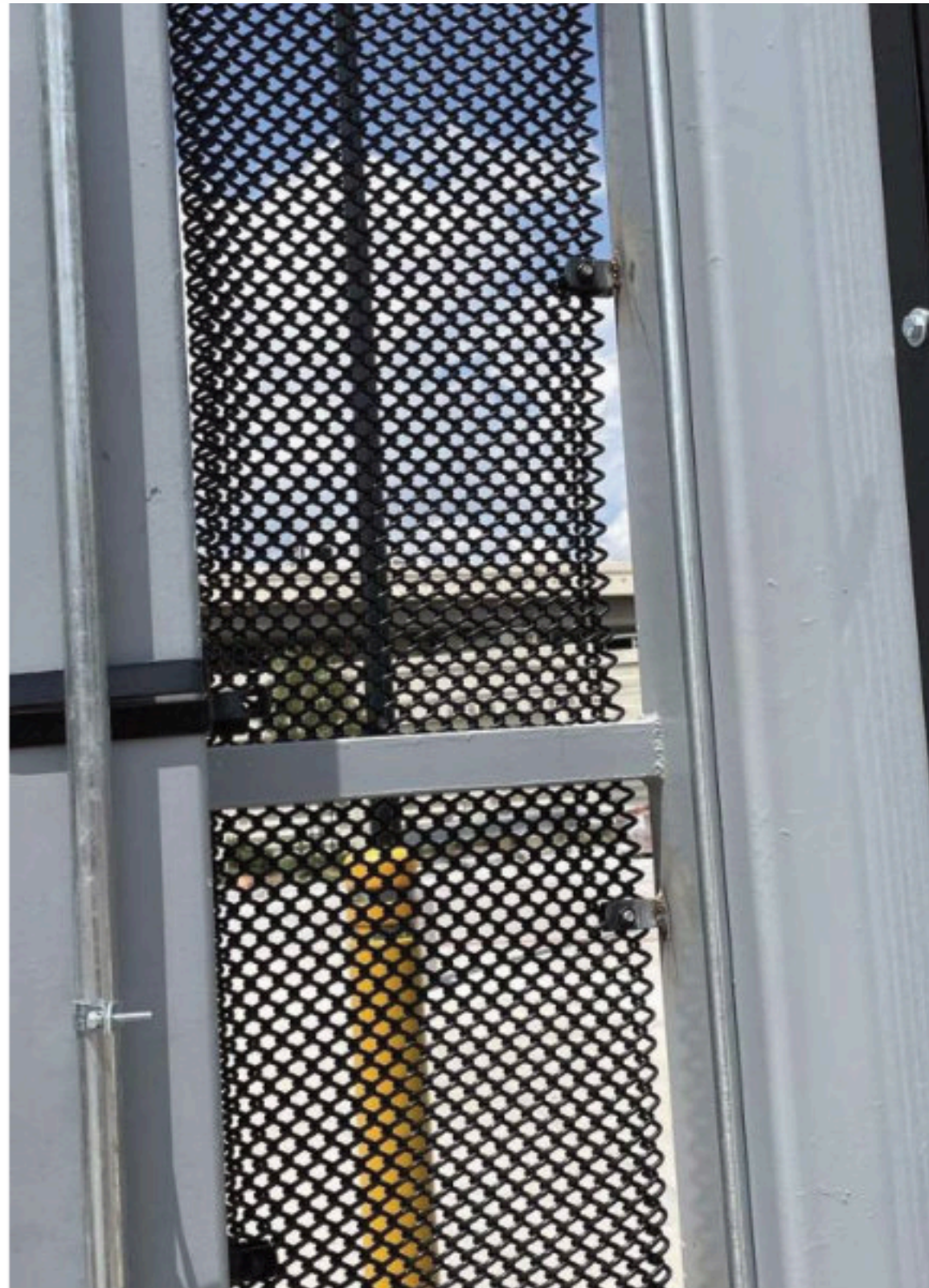
FNC-2- Enlargement of Black Expanded Metal Mesh Fence: To Be Located behind Vertical Metal Fence
